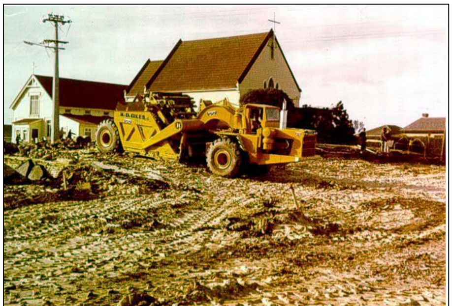
Road works for Highbury by-pass - beside Zion Methodist Church 1970's
