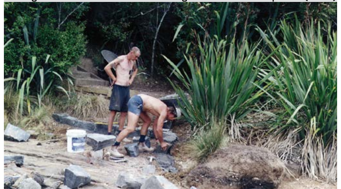
Making use of stone found on site to protect the midden
