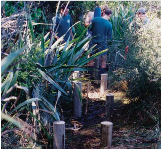
Pile driving for boardwalk
