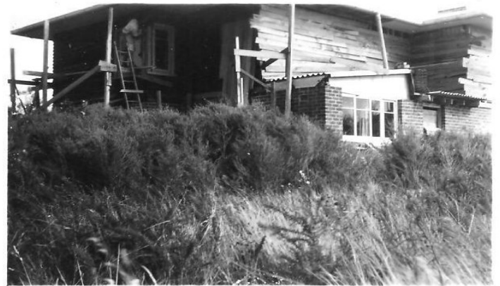
Construction continues, roof in place. Bach still visible below.
