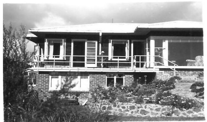
Completed - doors opening from 2 bedrooms, the bach now a small flat below, next to a garage. Lounge windows R) overlooking the sea from above cliffs at Campbells Bay. Today – two townhouses now fill the space.
