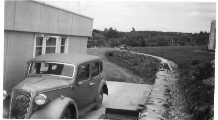
Campbells Bay bach, with retaining wall beside the drive.
